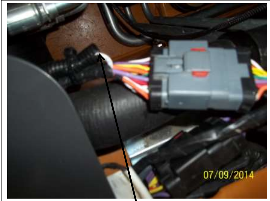
New wire connection secured in place
