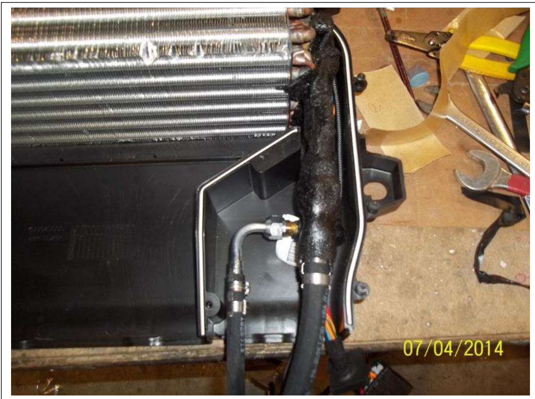
Set coil into place and the re-install the lid
