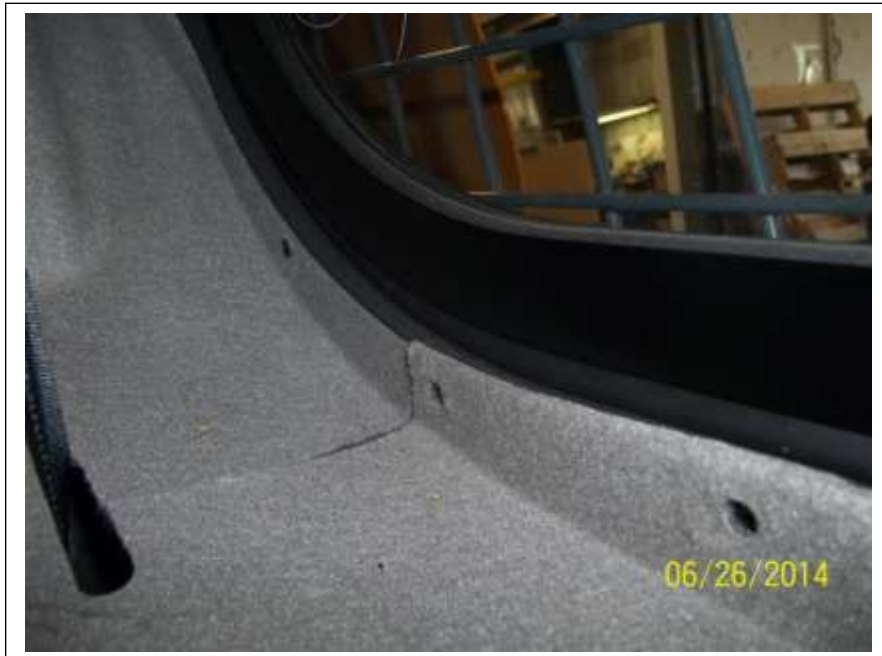
Removing button clips to get access to the heater box.
